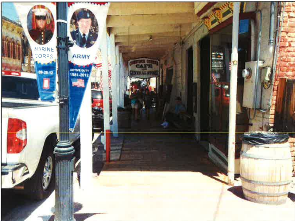
Figure 6 – Site Photo (looking north along boardwalk)
