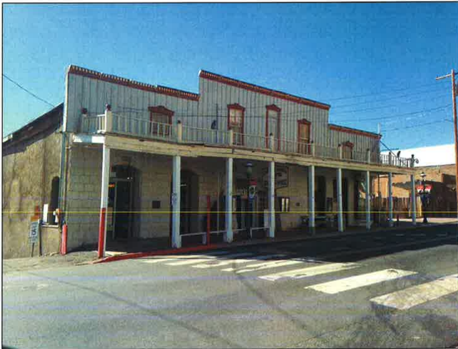
Figure 4 – Site Photo (front)
