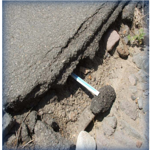
Erosion actually extends under the road and more pieces will break off.
