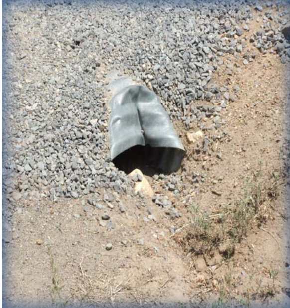
Crushed and debris filled corrugated pipe opening.
