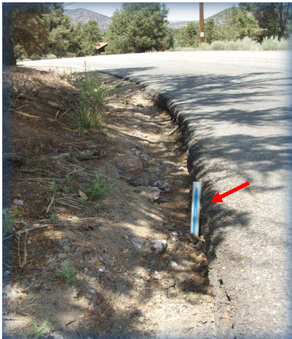
Red arrow points to a 12" ruler. Drop-off is almost 12" on the road edge and considered a safety issue by NDOT.
