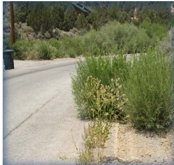
Examples where larger vehicles are forced to drive through vegetation when two vehicles meet on the road.
