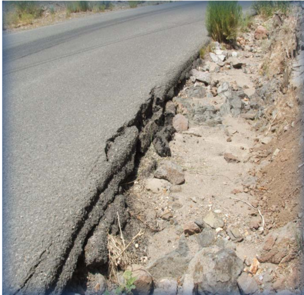
Road is breaking off in pieces.
