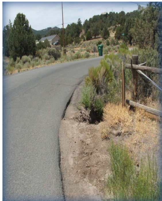
Hole is scoured out near edge of roadway.
