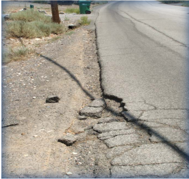
Drainage runs along edge of road rather than in the ditch a few feet away.
