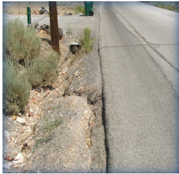
Drainage along road edge eventually ends up flowing back into ditch.
