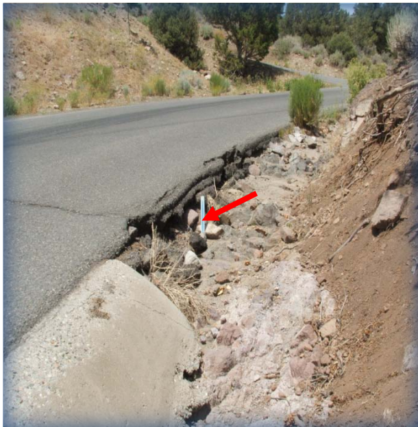
Red arrow points to a 12" ruler. Drop-off is 12" on the road edge and considered a safety issue by NDOT.
