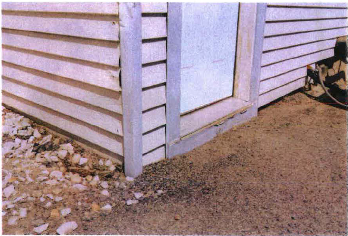
FIG 7 Exterior view of threshold at rear door with siding at grade
