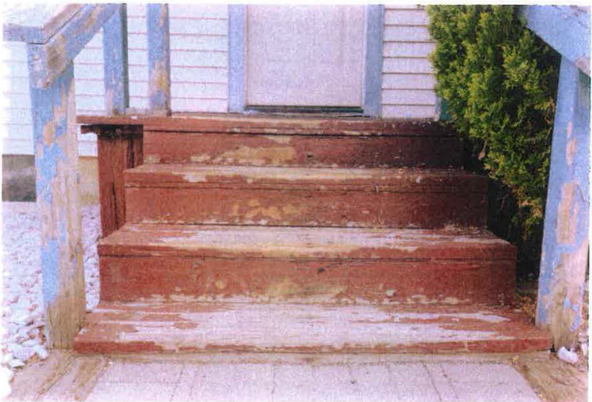
FIG 10 Exterior view of front steps. Non-compliant first riser
