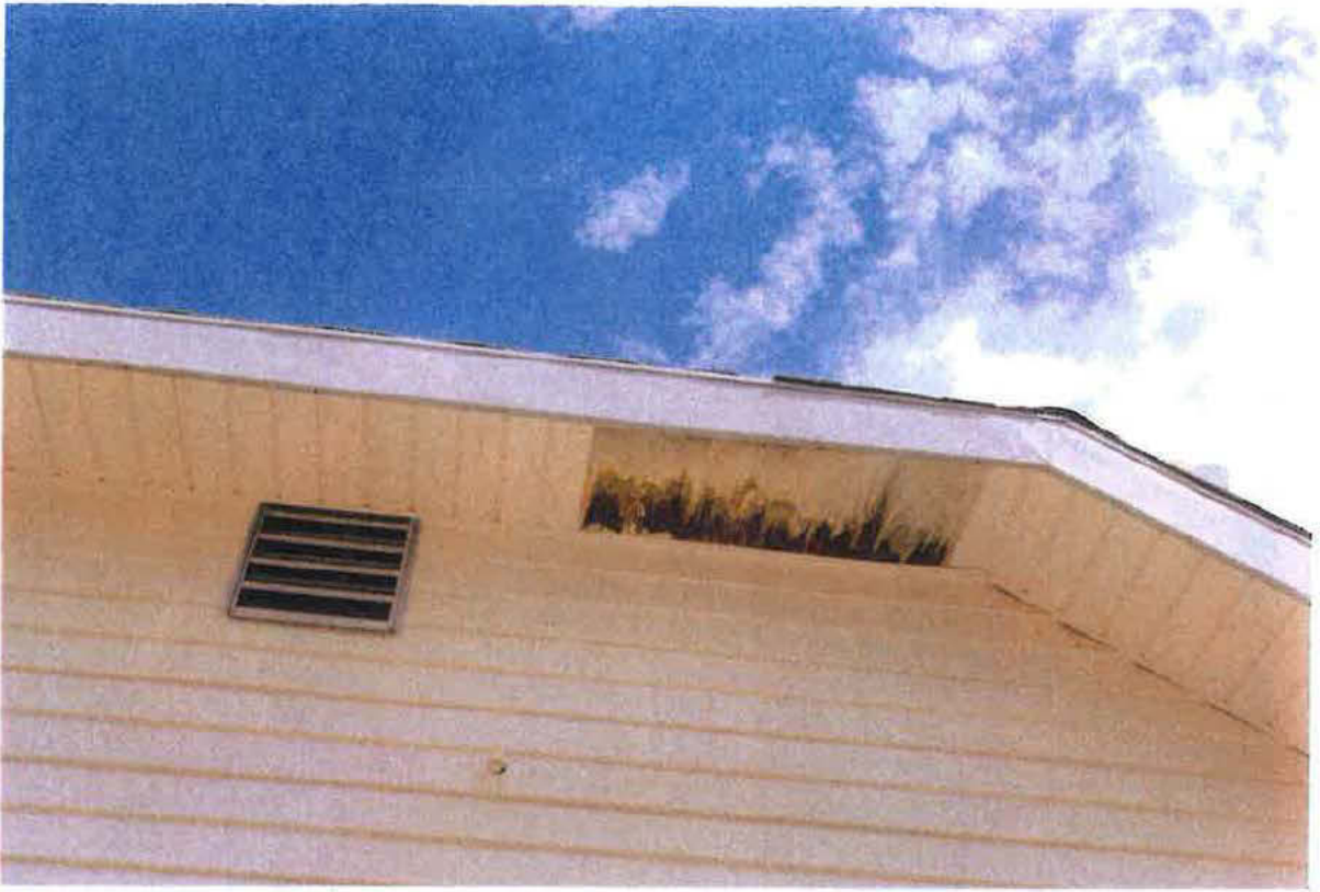
FIG 9 Exterior view of water damage at soffit
