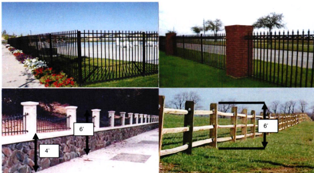
Figure 12.5: The wrought iron fences (top) are easily seen through by adjacent vehicular and pedestrian traffic and are considered see-through fences for the purpose of this section . The top left fence, with no large supporting columns, may be located within the vision-clearance-triangle; the top right fence, with vision obstructing columns, may not. The 6 foot fences (bottom) may abut the front lot line of the E, and R zones because the solid portion meets the is at or less than the maximum height limitation for fences and walls in the front yard even though the entire fence is over the listed height limit . The bottom left fence/wall combination, like the top left fence, employs large support columns and must be placed outside of the vision-clearance triangle.
